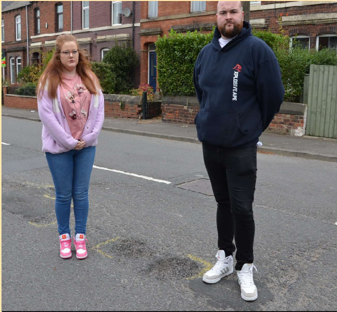
●Lauran Sowerby and Joe Sowerby on Station Lane where resurfacing is to take place.
