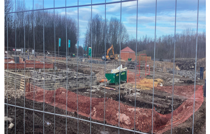
New Housing in Progress
